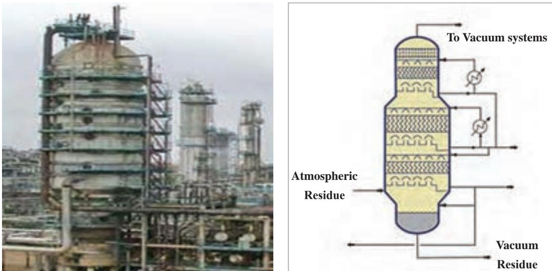
Fig. 20: Vacuum distillation tower
