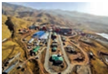
Gold processing plant
