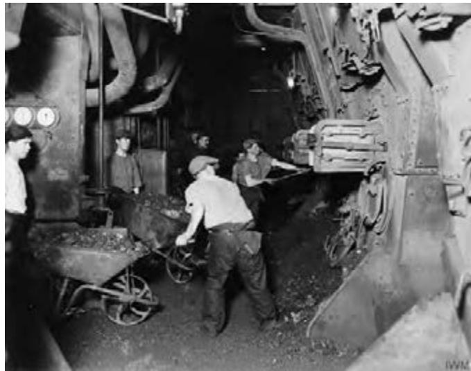
Steam ships boiler room
