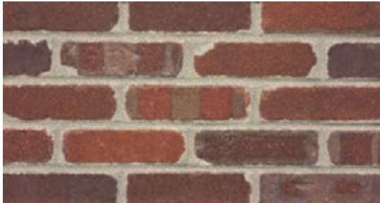
Standard 3/8" Mortar Joint
