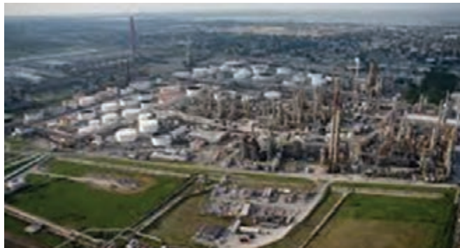
Fig.9: A chemical plant
