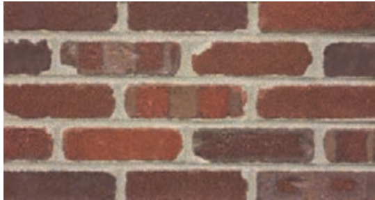
Standard 3/8" Mortar Joint
