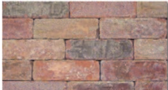
No Mortar Joint (Dry-Stacked)
