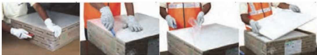
Wrong box opening method
