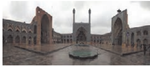
Jame Mosque of Isfahan ▲
