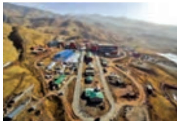
Gold processing plant
