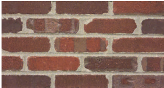
Standard 3/8" Mortar Joint
