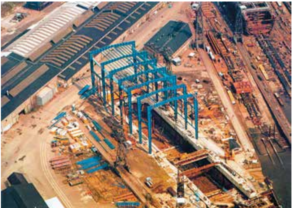
Covered graving Dock "D" during construction
