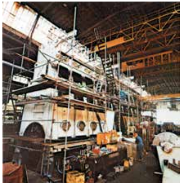
Assembly of a main Diesel motor
