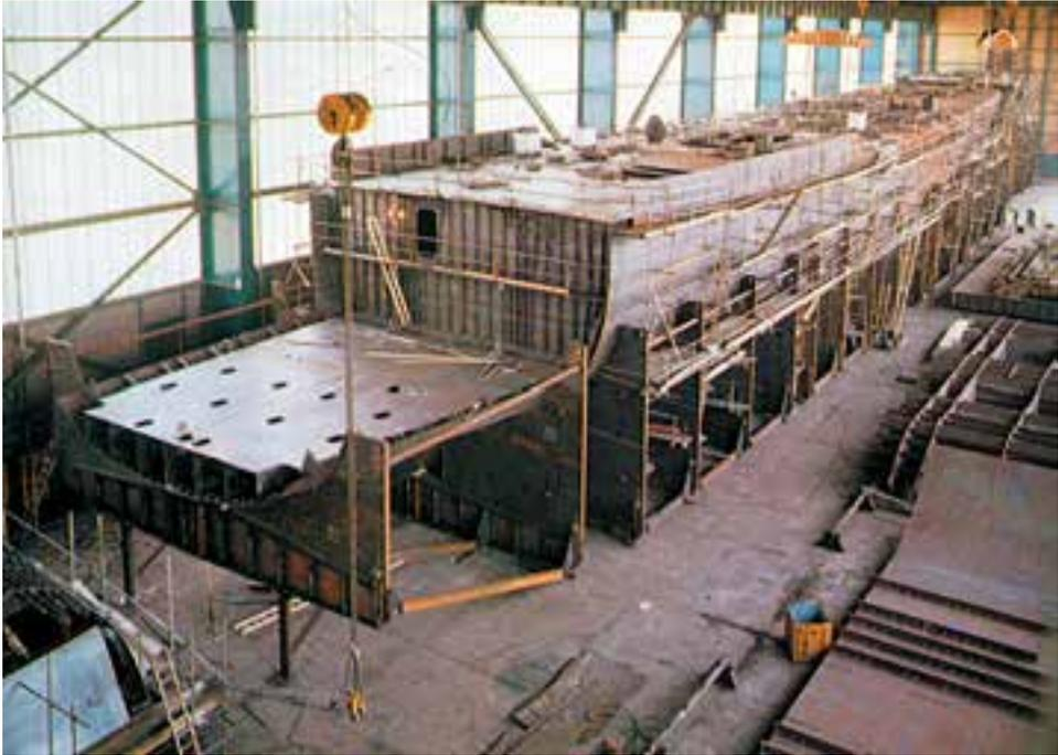
**No. 1 Frigate under construction in Assembly Hall**
